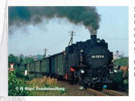
Since the German State Railroad still needed class 99.73-76 locomotives spread across Saxony, several of these locomotives were updated towards the end of the Sixties. On the one hand they were given a general overhaul, on the other hand — and that was immediately visible — new water tanks and coal bunkers were added which were welded instead of riveted.
